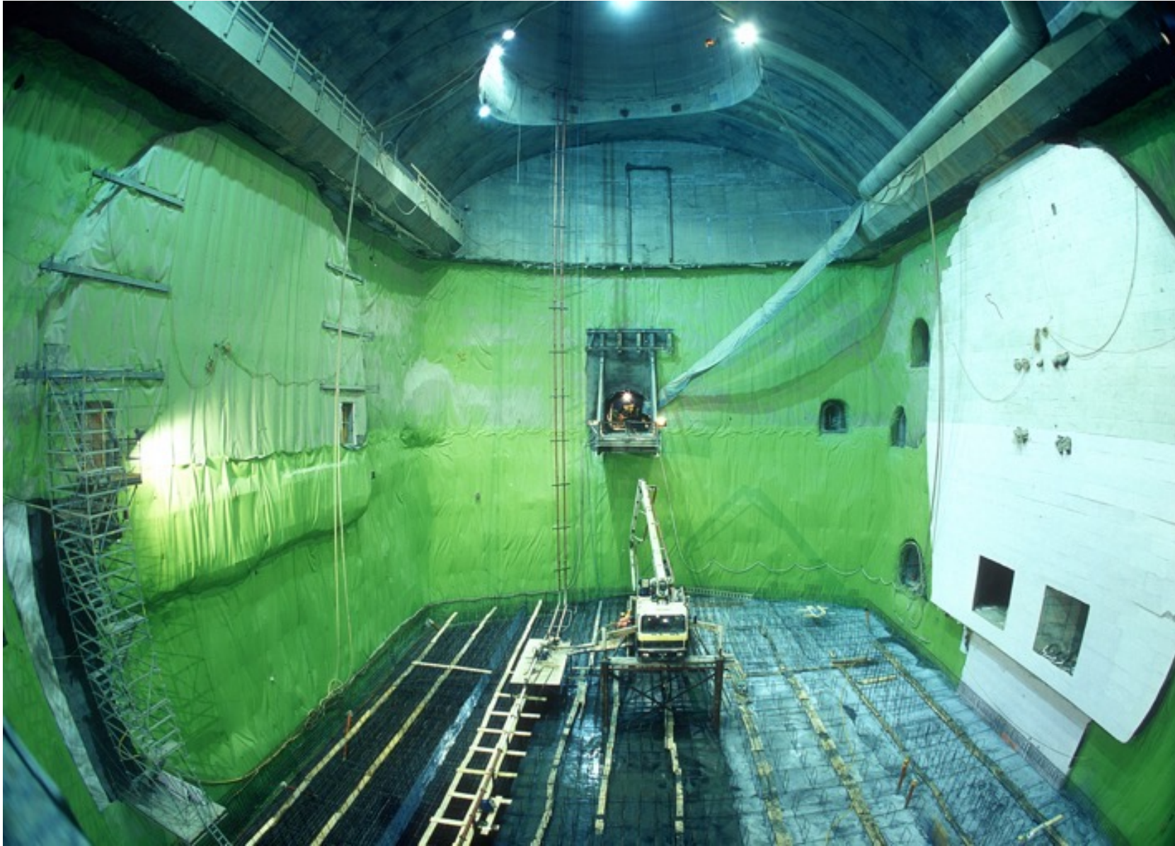
ATLAS cavern after excavation in July 2002
