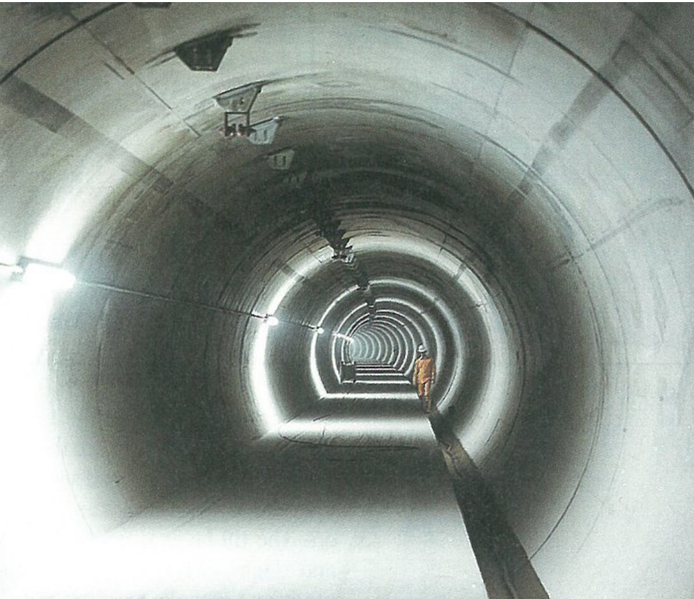
LEP tunnel before installation of bending magnets
