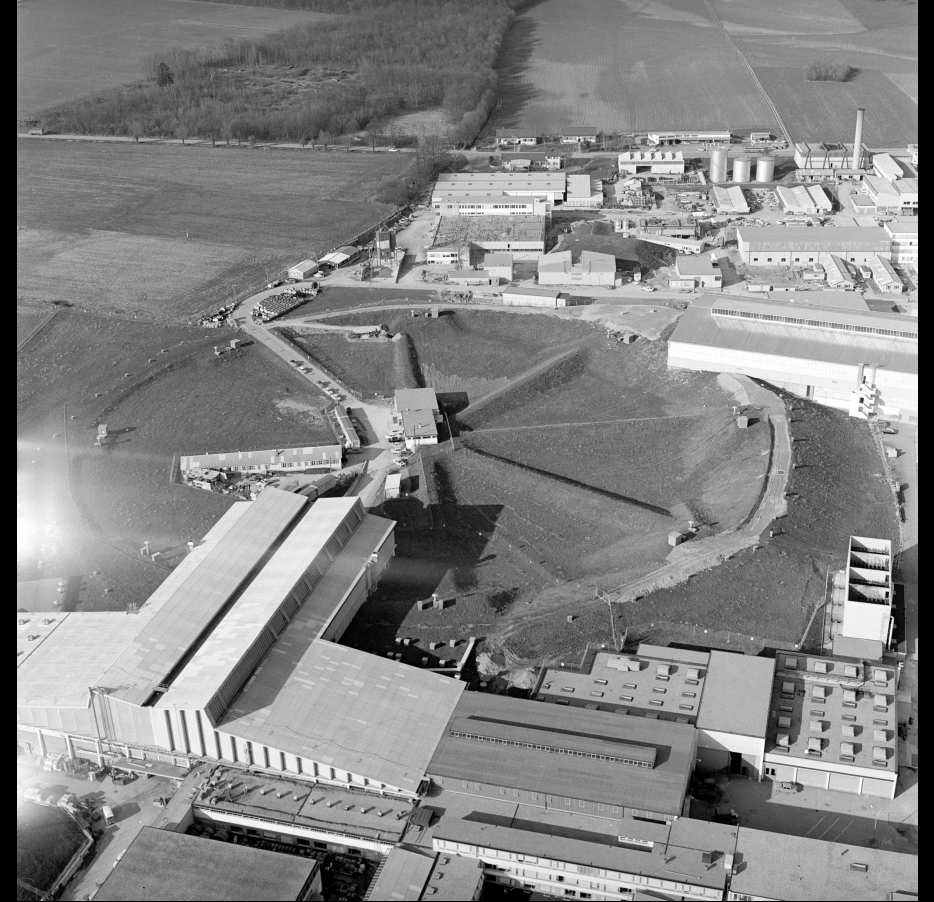
Aerial view of the 25 GeV Proton Synchrotron at CERN in 1965
