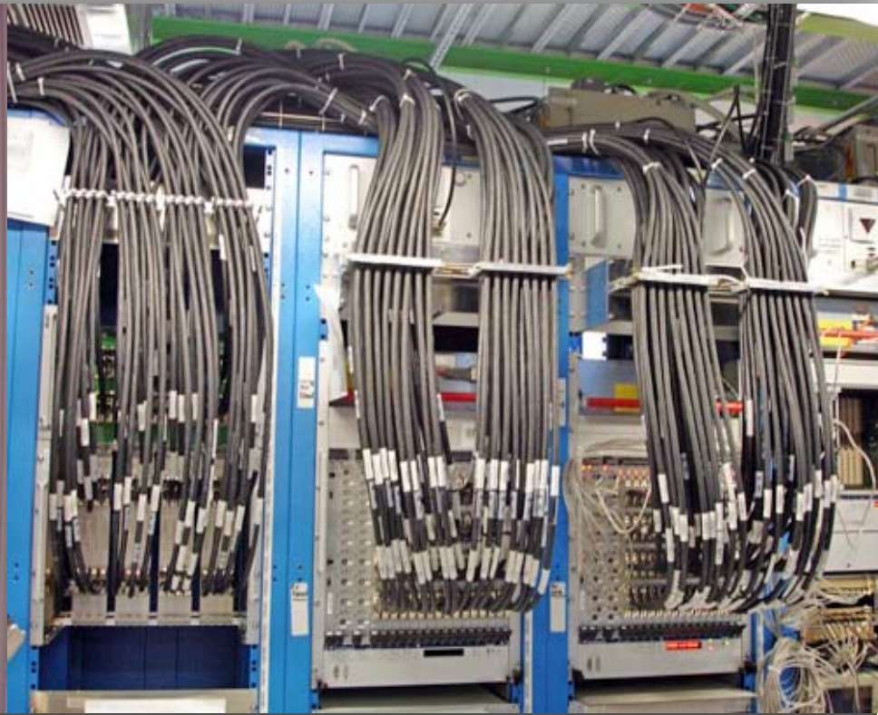
Analogue trigger cables received in electronics cavern
